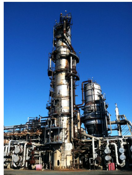
Atmospheric Crude Tower
